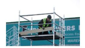
13. Fit the toeboard clips to the rung next to the corners of the platforms and then fit the toeboards as shown.
