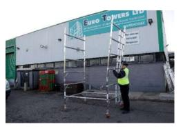
4. Fit the next set of frames onto the base, ladder frames run continuously up the left hand side. **Note:** see kitting page for frame
