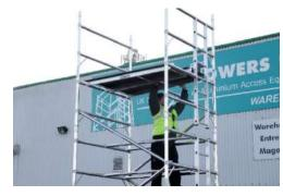
11. Fit the plain platform followed by the trapdoor platform 4 rungs above the one you are standing on. **Note:** There must always be 2 rungs clear above any platform so you can fit safe guardrail braces.
