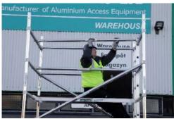
8. Climb the ladder inside the tower and sitting through the trapdoor fit 4 horizontal braces face down onto the 1<sup>st</sup> and 2<sup>nd</sup> rung above the platform to form your guardrails, as shown.
