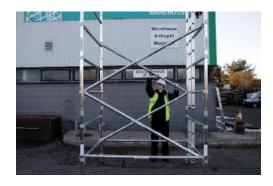
5. Add 4 diagonal braces from the  $1^{st}$  to  $3^{rd}$  and  $3^{rd}$  to  $5^{th}$  rungs as shown, level the tower using a spirit level as a guide.
