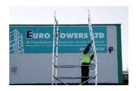
9. Standing on the platform, add a set of 4 rung frames, ladders run in a continuous pattern.
