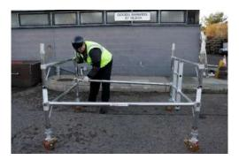
3. Fit another horizontal brace on the ladder side of the frames face down onto the 1<sup>st</sup> rung. Note: when standing inside the frames looking at the ladder frame, the ladder should be to the left hand side.
