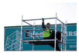
12. Climb the ladder inside the tower and sitting through the trapdoor fit 4 horizontal braces face down onto the 1<sup>st</sup> and 2<sup>nd</sup> rung above the platforms to form your guardrails as shown.
