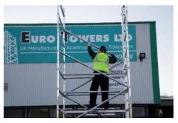
10. Add diagonal braces continuing the pattern from the previously fitted braces.
